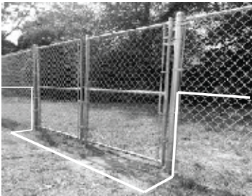
Bury cable in front of gates and use right angles when positioning to the fence.
